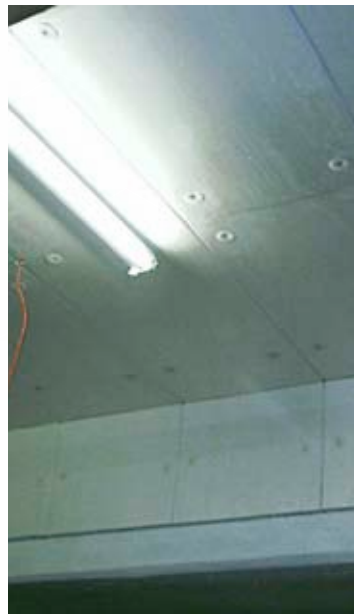
IsoBoard Under Soffit: Exposed Parking Insulation
